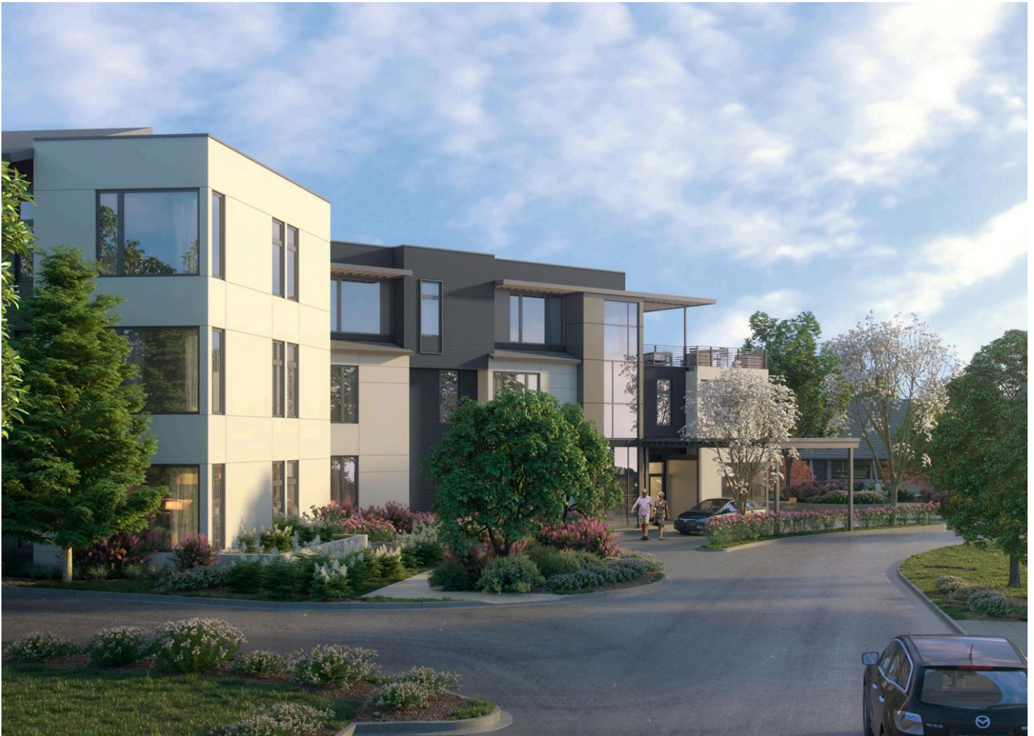
Mount Calvary Senior Living will be an all-electric design, an important piece of Boulder Housing Partners' sustainability goals.
